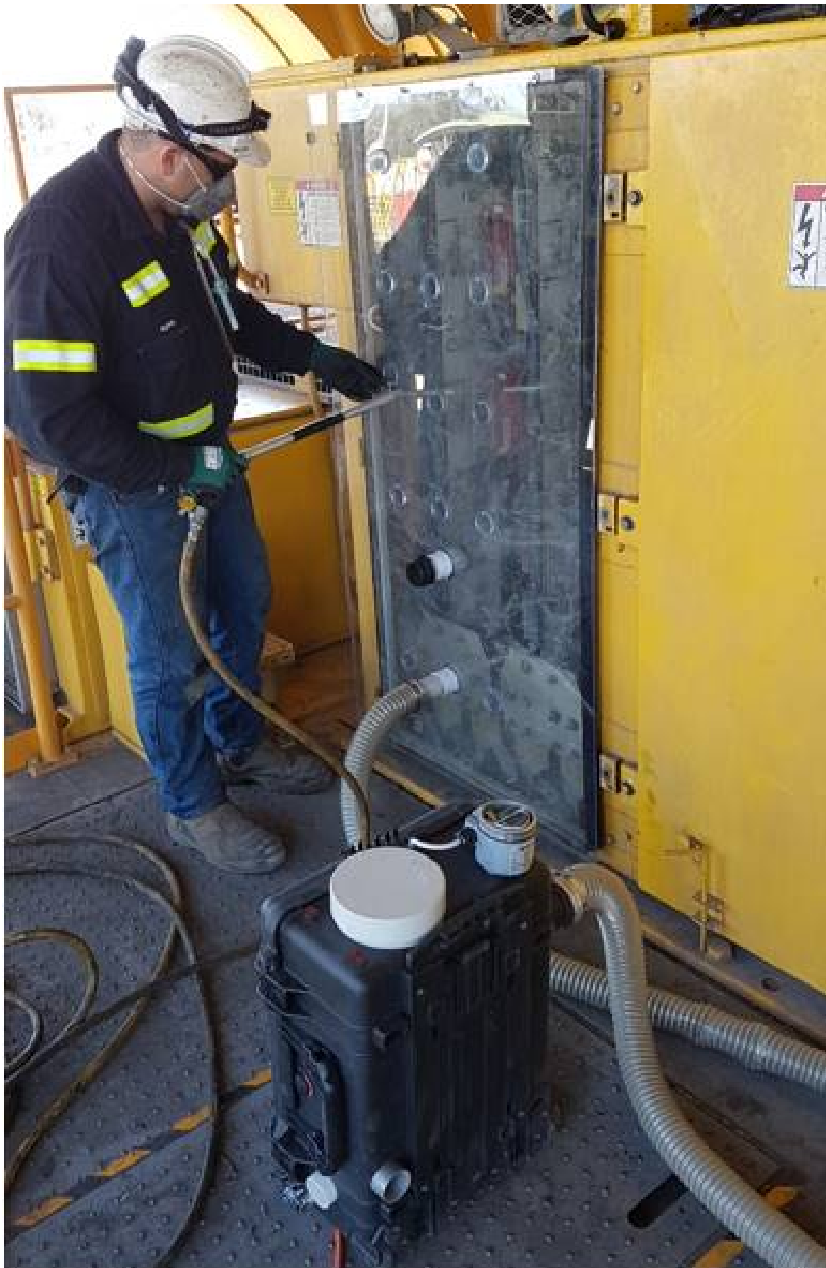
Figure 11. Blow-out cleaning with a prototype containment cover and prototype Plev
