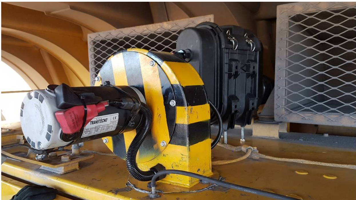
Figure 10. Pressurisation fan on top of cabinet, and the inlet filter can be seen behind the fan.
