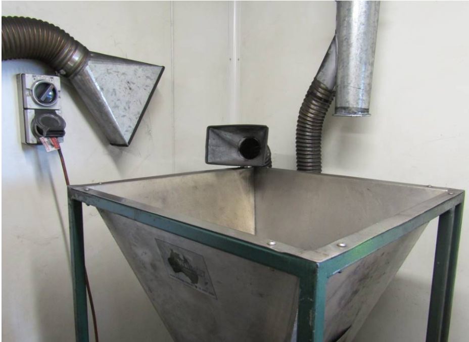
Figure 5. Example of movable and adjustable LEV's in a coal laboratory to account for dust sources (LEV's held in position by magnets)
