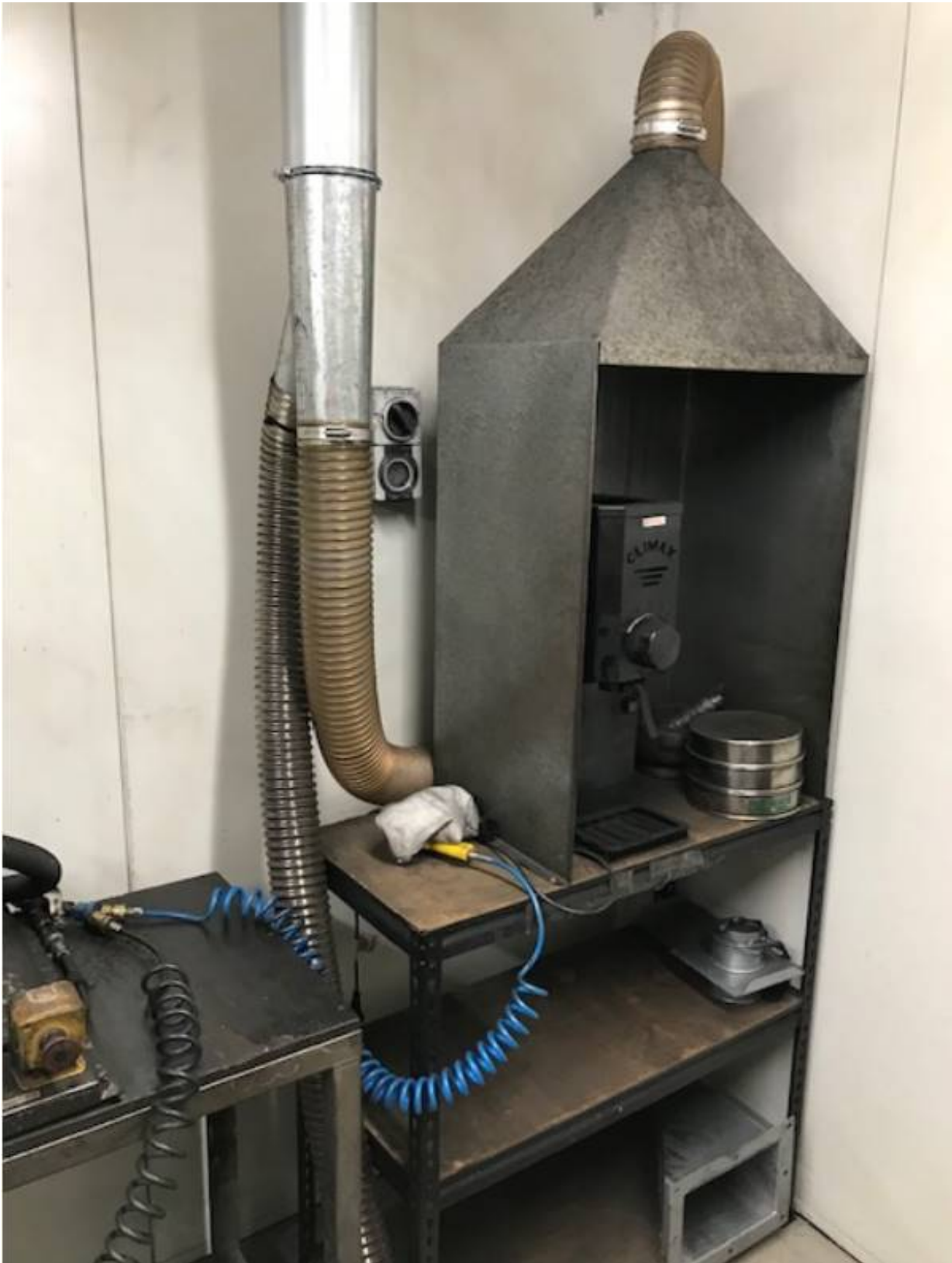
Figure 7. Example of a fixed LEV system in a coal laboratory
