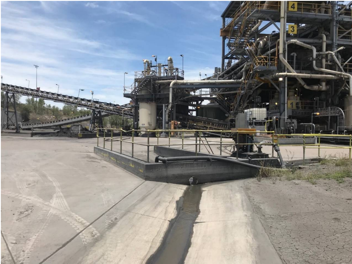
Figure 1. Concrete aprons below and around CHPP with drainage leading to sumps
