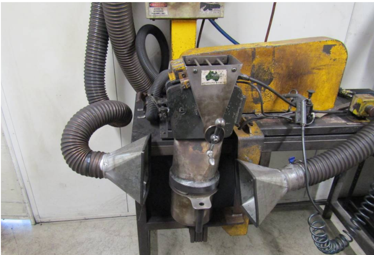
Figure 6. Example of a LEV system in a coal laboratory. Movable and adjustable LEV's to account for dust sources (LEV's held in position by magnets)
