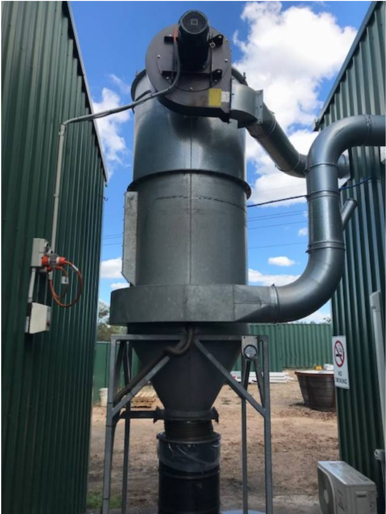
Figure 8. LEV system outside a coal laboratory with all dust collected in the bin at the bottom of the system
